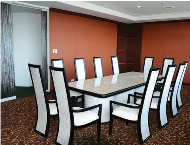
Construction refurbishment of the Presidential Lounge and Dignitaries Lounge, both of which were completed during the year, and the VIP Room whose completion is targeted in 2015.
